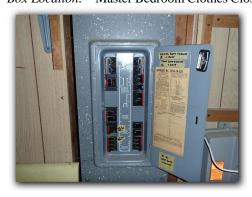
There is a Federal Pacific panel box in place at the time of the inspection. Due to the age of the panel box and the problems associated with this type of panel box, upgrading this panel box with a more current panel box is recommended. Full evaluation of this panel box is beyond the scope of this inspection. You are encouraged to have the panel box further evaluated by a qualified electrician *prior to closing*.
