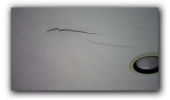
Water stains were observed at or around the water heater flue in the garage. The cause and remedy should be further evaluated and corrected as necessary.
