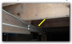
There was evidence of previous water penetration in the crawl space. This condition may vary seasonally. Water penetration may negatively affect the performance of the pier and beam foundation. Lot drainage improvements and/or the installation of a moisture barrier should be addressed as a first step to controlling water penetration of the crawl space. This condition should then be monitored to determine if other drainage improvements are necessary.
