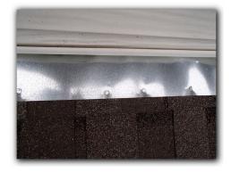
The roofing felt paper was observed to be installed under the lower metal drip edge flashing detail and in some places felt paper did not cover all of the decking. This may allow water to seep behind the fascia board and soffit/eave areas over time. Monitoring is recommended to determine if corrective measures are necessary or cost effective.
