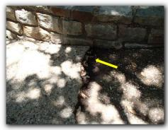
The elastic caulk (Deck-O-Seal or other brand) between the deck and coping was observed to be in the early stages of cracking. Monitoring is recommended.
