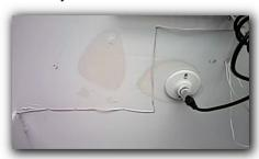
The ceiling of the attached garage adjacent to the living space was not fire taped at the joints or the fire taping is damaged or failing. Drywall cladding on garage ceilings and walls that are adjacent or common with the living space should have the joints taped and sealed to provide the required fire rating for attached garages.
