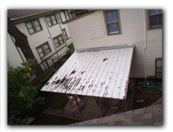
Roof fasteners (nails and/or staples) were observed to be exposed on various locations of the roof including the ridge caps and flashing areas. All exposed fasteners should be sealed with the appropriate roofing caulk or sealant.
