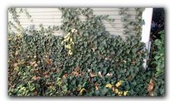
The wood siding and wooden supports were making wood to ground contact by design. This condition may promote wood rot and may attract wood destroying insects. These areas should be monitored and corrective measures taken it necessary.
