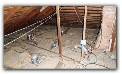
The insulation was inadequate. Adding insulation to a minimum depth of nine inches is recommended.
