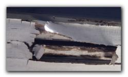
The wood siding and trim was observed to be damaged or deteriorated at the north, east, west, and south sides of the house, particularly along the lower edges of the siding. Repair is recommended.
