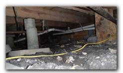
One or more of the piers were not touching the beam or floor joist. Shimming or other repairs are recommended.
