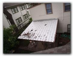
Roof fasteners (nails and/or staples) were observed to be exposed on various locations of the roof including the ridge caps and flashing areas. All exposed fasteners should be sealed with the appropriate roofing caulk or sealant.
