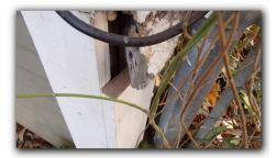
There were openings in the exterior veneer in various locations including at the north and east sides of the house that need to be sealed to prevent water or pest intrusion into the crawlspace.
