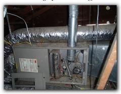
The heating equipment appears to have reached the end of its serviceable life expectancy.
